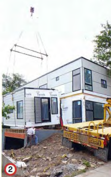
1. After more than a year of delays, delivery at last. The crane carefully lowers the second-floor “box” onto the first-floor den, and living and dining rooms. 2. The kitchen and foyer module is set in place over the tuck-under two-car garage. 3. Schmit’s finished 2,010 square-foot home.
